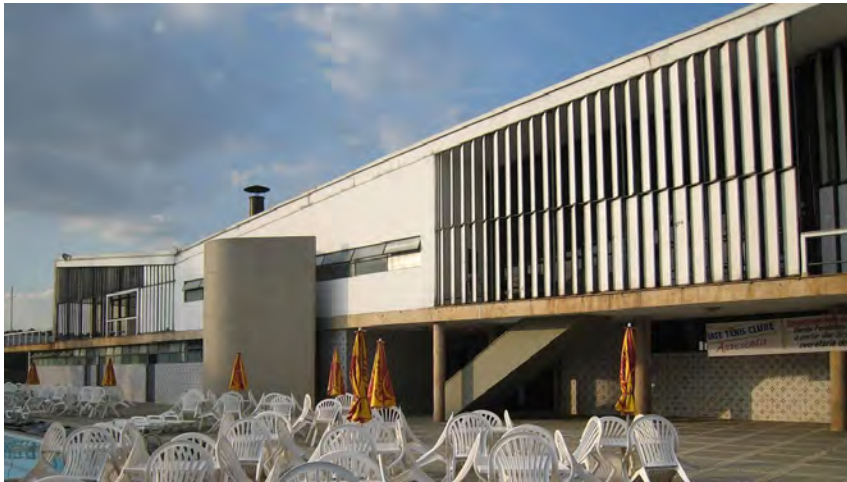
4: Terrace to the left and large glass panels with brise-soleil to the right. Photo: Shelley Bernstein.
