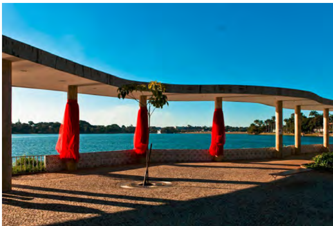
14: Casa do Baile, canopy framing the view. Photo: Cristiano Maia.
